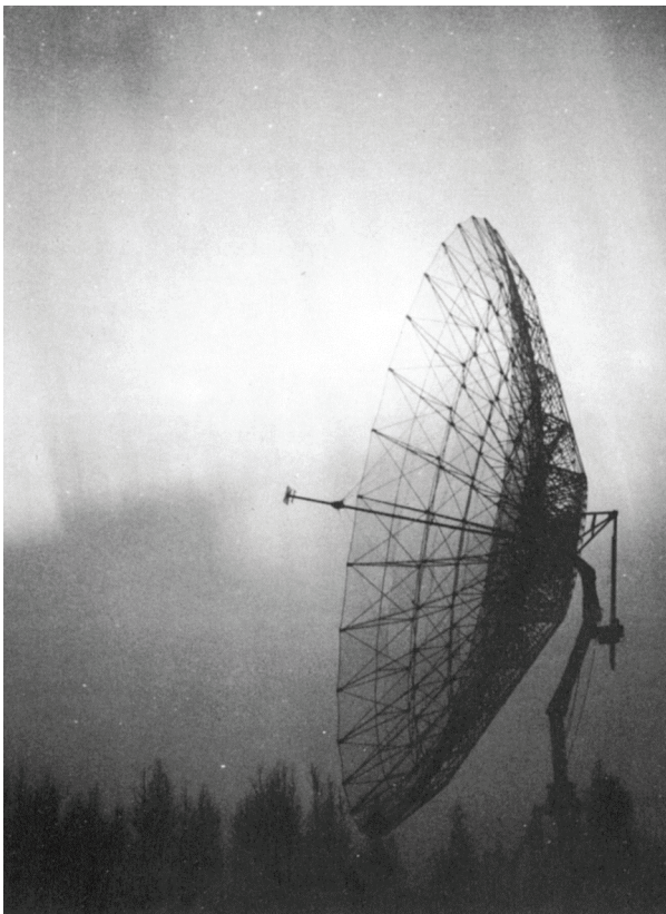
Figure 9-3. SRI’s 60-ft. auroral radar located just outside Fairbanks AK (visual aurora in the background).
